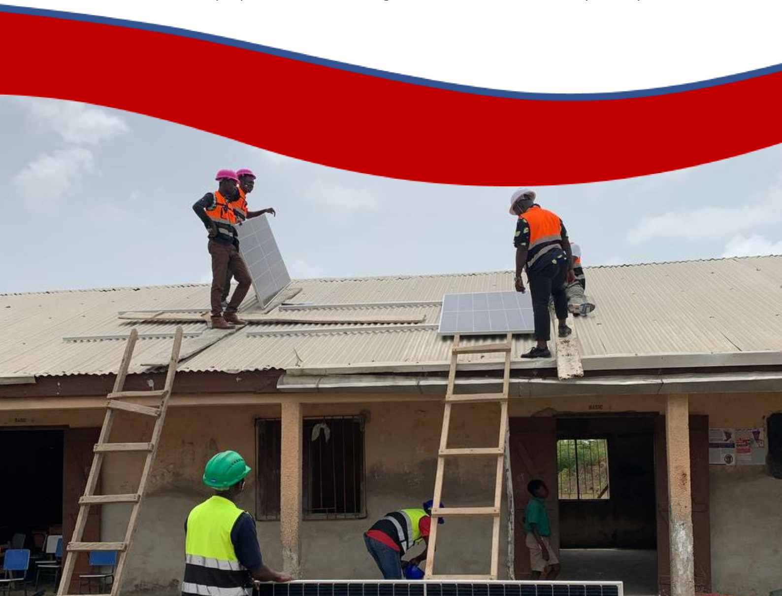
Our volunteers and Trainees installing the solar power system
